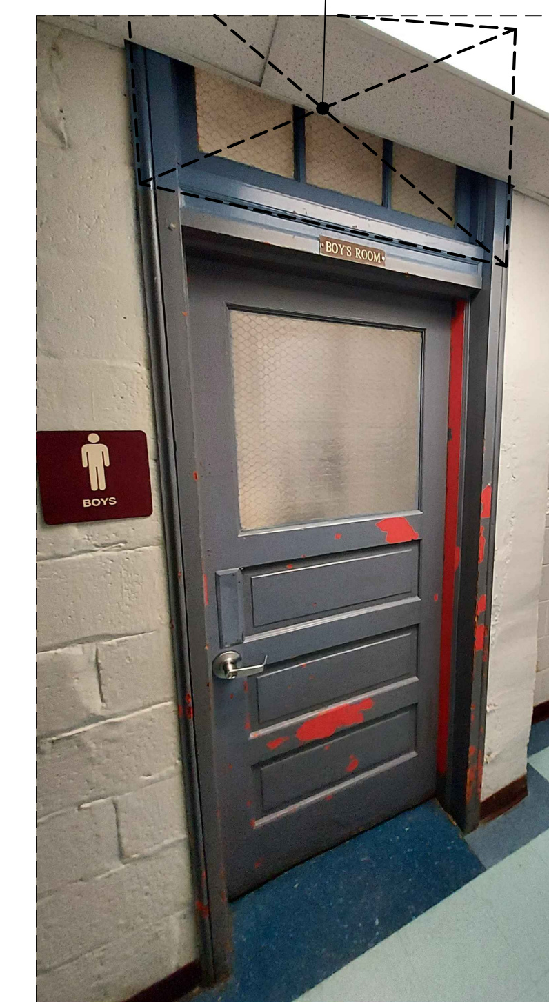
EXISTING DOOR NOTE: COMPLETE DOOR, FRAME AND TRANSOM TO BE REMOVED
